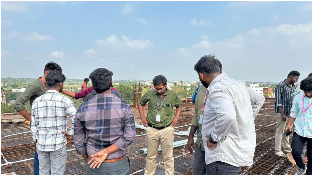
Industrial Visit to MVR Cinemas Construction Site, Guduvanchery on 31/1/2024
